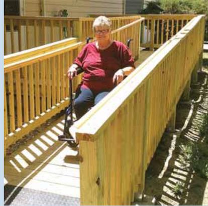
Examples of eligible modifications include outside ramps and lifts, grab bars, handrails, widened doorways, accessible tubs and showers, and reachable sinks and counters.
